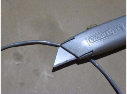
Hold the blade perpendicular to the cable, and draw it across the cable lightly as you rotate the cable along its long dimension. This creates a scored line through the plastic jacket. With a sharp blade, not much pressure is needed. You may need a bit of practice to get the feel.
